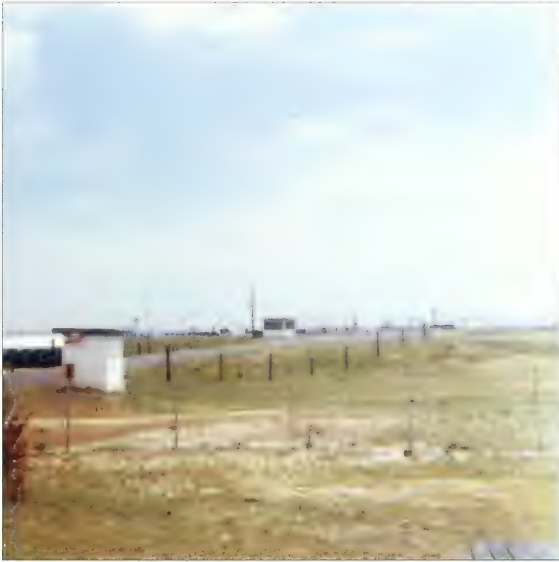
Figure 5.112. View looking northeast at the missile magazines, NIKE launch site, circa 1968. The vehicular connection between the Ready Barracks and the Missile Magazines and Missile Maintenance Area to the east was maintained on either side with a turf mixture (GATE 22041).
